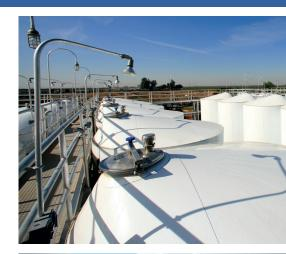
"The insulation on the tanks allows us to quickly chill and easily maintain the optimum wine temperature in any weather. Due to the fact that we insulated approximately 20% of our outside tanks each year, over the last five years, we have experienced a noticeable reduction in our PG&E bill for the same time period."
